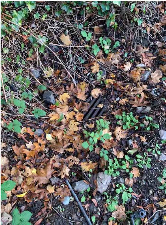
Catch Basin at Point I
