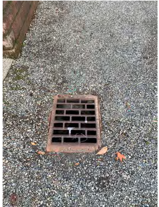
Catch Basin – Point C
