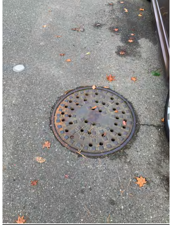
Catch Basin at Point F
