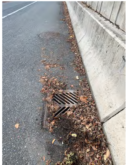
Catch Basin At Point O -Far Side
