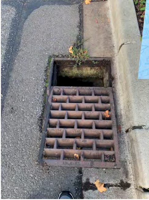
Catch Basin At Point L
