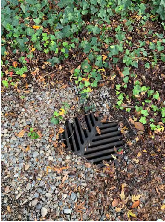
Catch Basin at Point H
