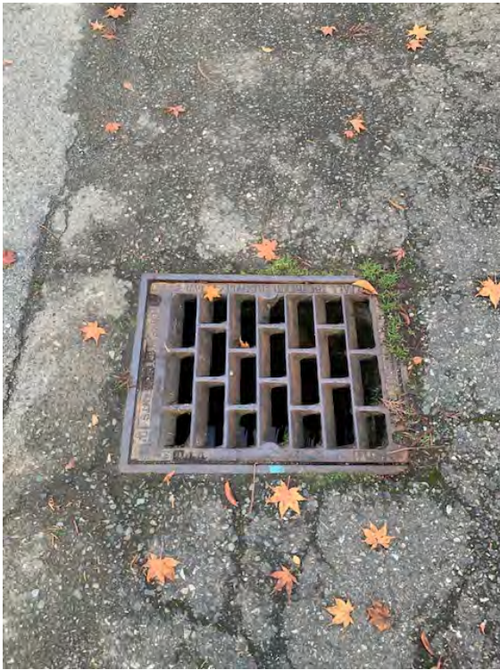
Catch Basin - Solid grate at E
