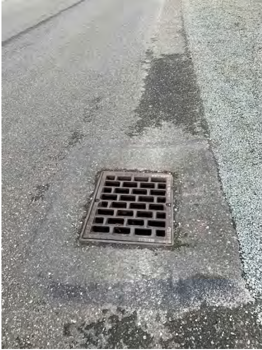
Catch Basin – At point A, Looking Downstream
