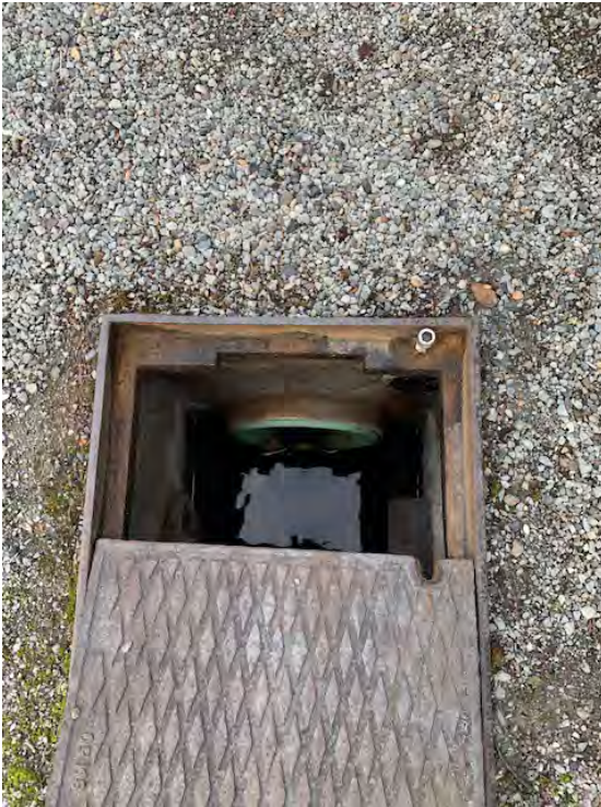
Inside Catch Basin – At Point B
