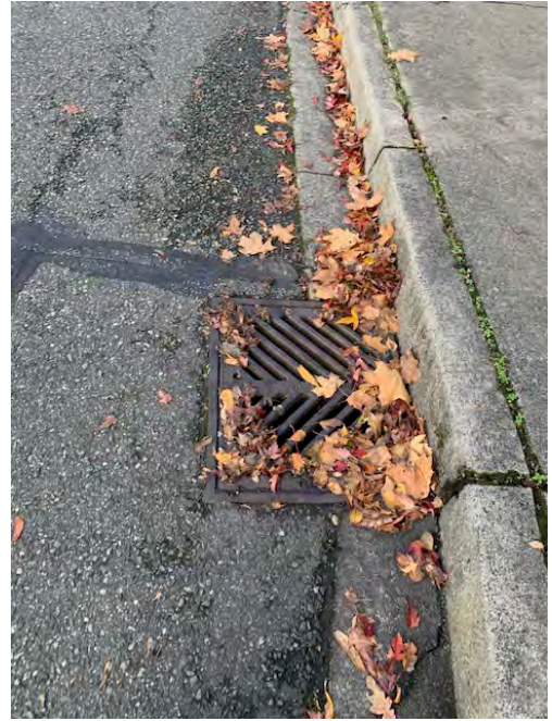
Catch Basin At Point N
