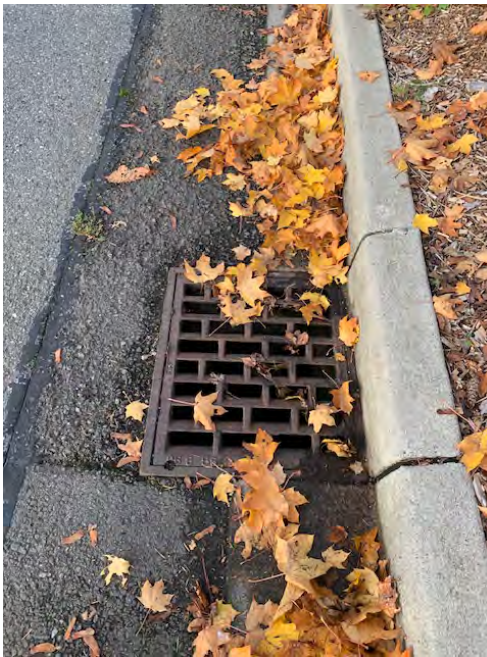
Catch Basin At Point M
